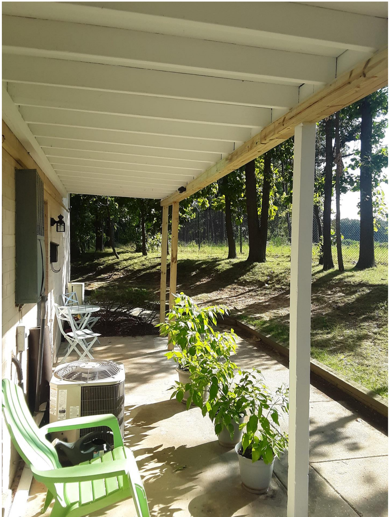
Aug 24,2022 – 3 pictures of 11412-105-106 porch - newly painted ceiling – new support
